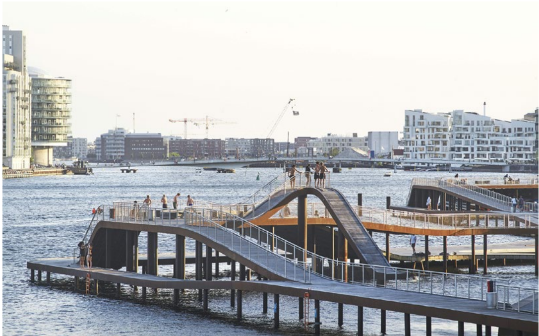
Kalvebod, Copenhagen, boardwalk
